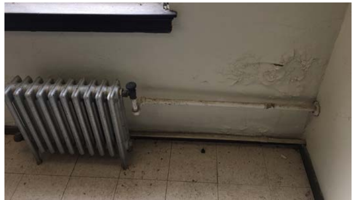
Asbestos floor tiles, water infiltration and outdated heating
