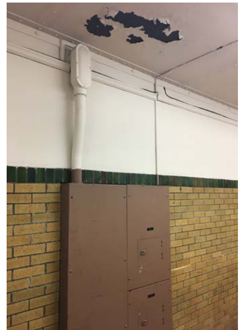
Ceiling paint peeling
