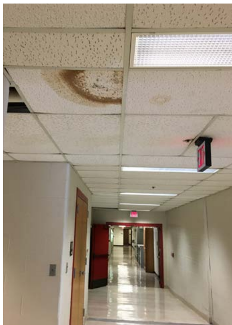
Water issues, leaky pipes, and condensation affecting ceilings
